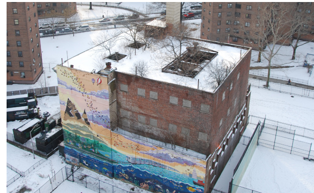
Baruch Houses, abandoned bathhouse, 2015
