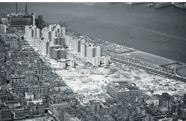
Low East Side, Jacob Riis & Lillian Wald Houses under construction, 1948
